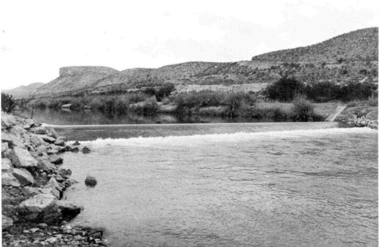
A five-foot weir at the Foster Ranch gaging station, immediately downstream from the Terrell-Val Verde County line.
